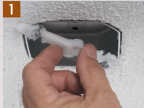
Back the screws out enough to slip the bracket on.
