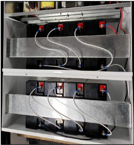
Battery brackets installed on the front
