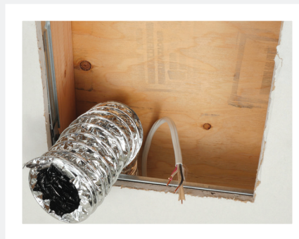
Existing 3" duct and wiring
