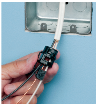
Feed cable through the knockout, then into the connector.
